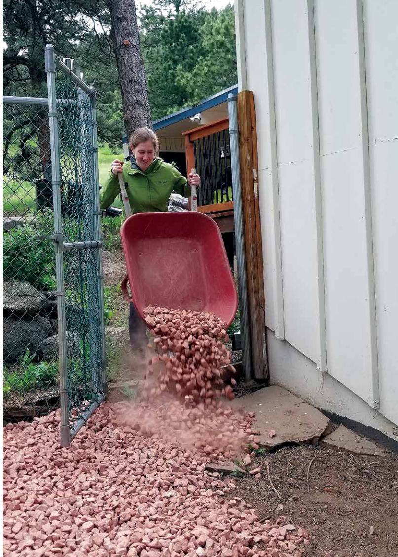
Top right: Preparing your home for wildfire can be accomplished as weekend projects, such as clearing vegetation from around your home's perimeter and adding noncombustible material near the foundation that won't ignite if embers land there. Photo: Wildfire Partners
