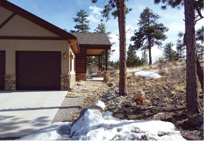
Top left: Hardening your home can include choosing noncombustible building materials like stucco paired with a stone facade. This house near Salida shows you don't have to sacrifice curb appeal to reduce the ignitability of your house. Photo: CSFS
