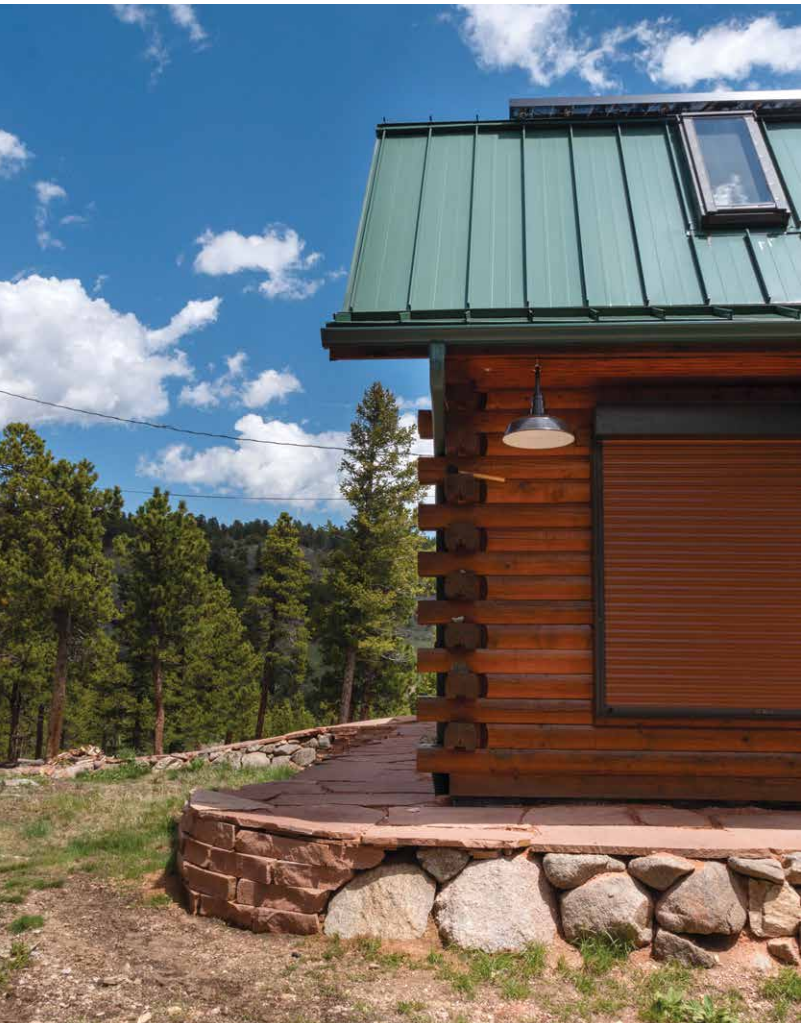
Bottom: A metal roof and noncombustible exterior window coverings add layers of protection against wildfire, in addition to the well-maintained defensible space that surrounds this home. Photo: Wildfire Partners
